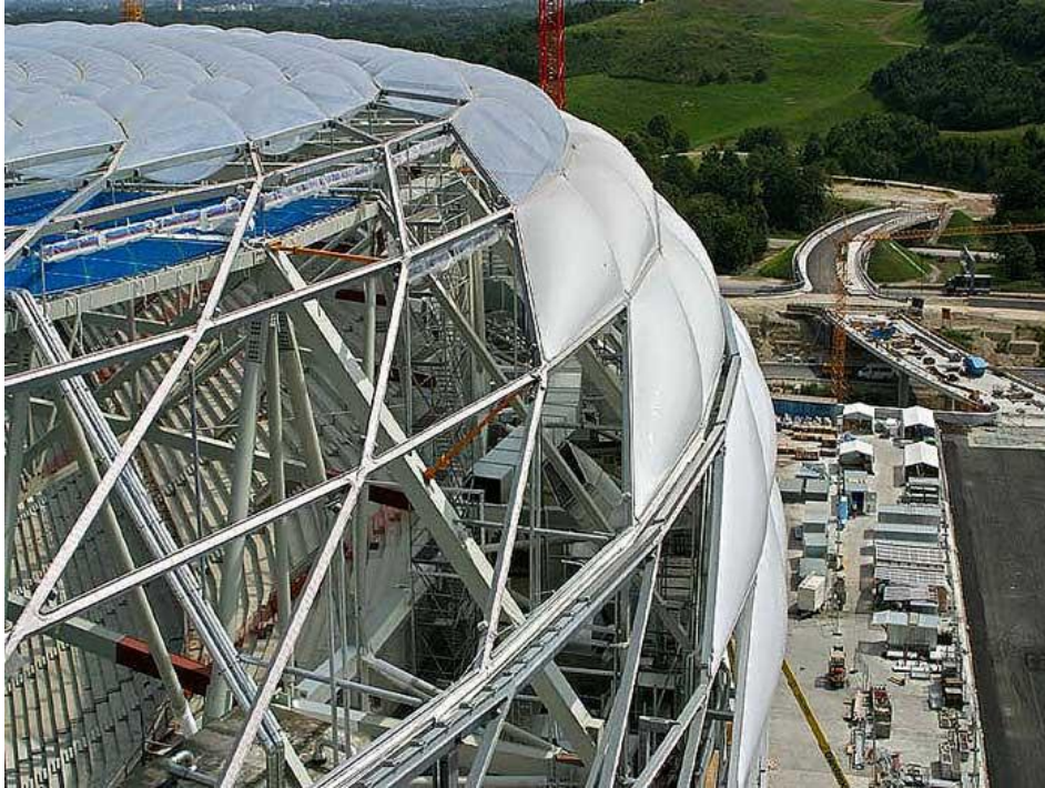
Figure 17 –ETFE membranes are fixed on metal grid.
