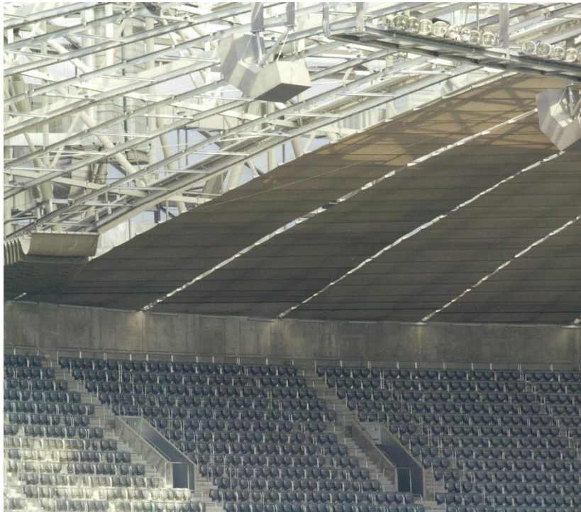
Figure 21 – Retractable ceiling extended.
