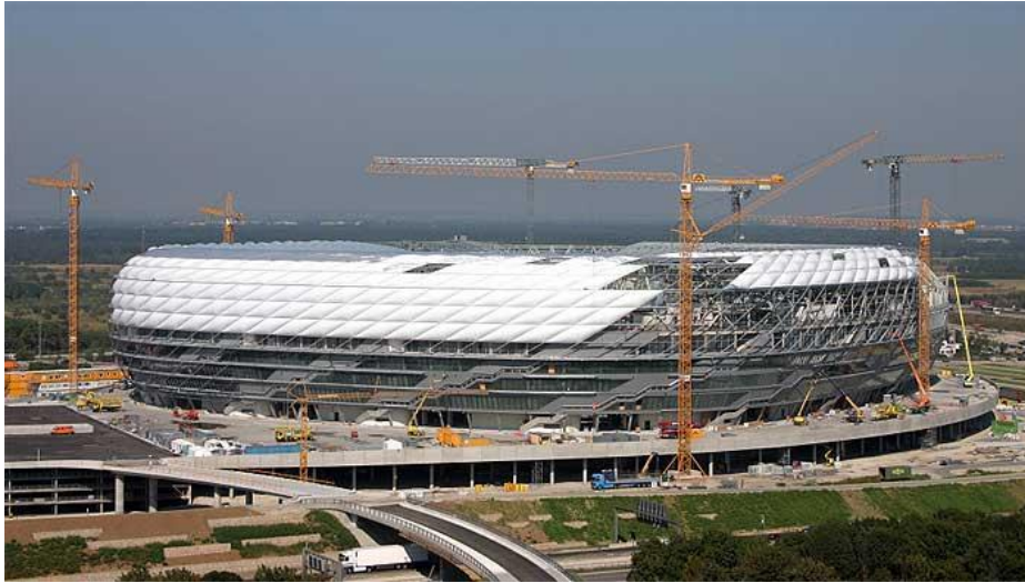
Figure 19 – Membrane attachment stage.
