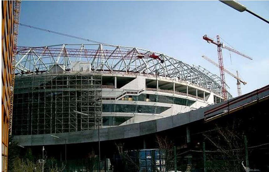
Figure 16 – Cranes raise up the metal trusses to 50 meters high.
