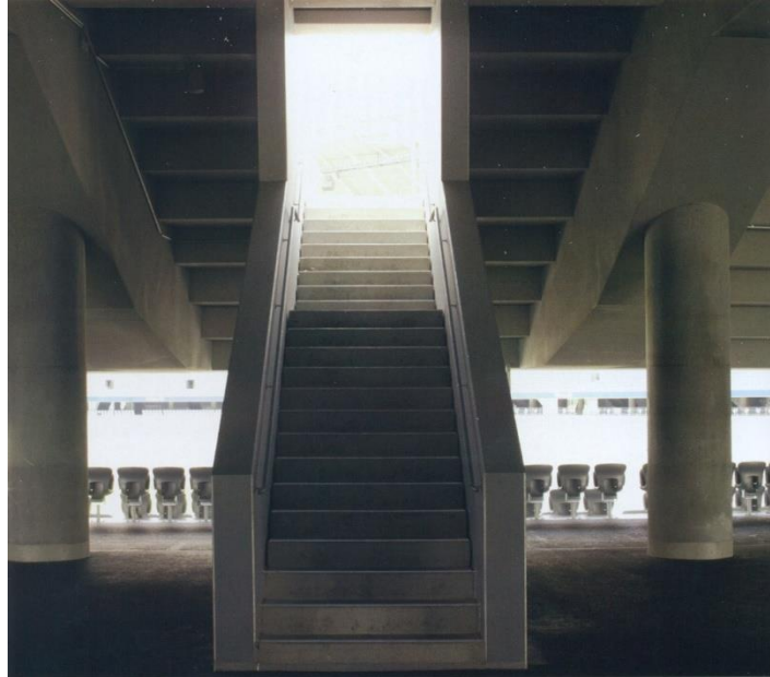
Figure 13 – Access stairs to the grandstands.
