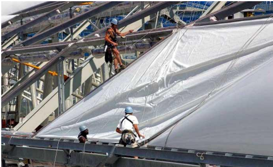
Figure 18 – Workers at 50 meters high install the membranes.
