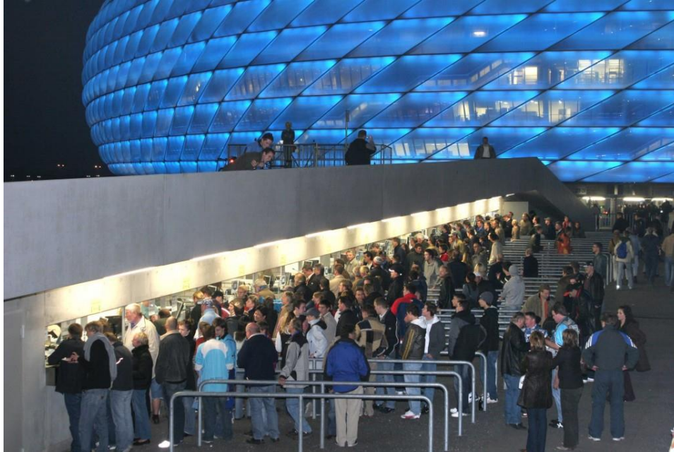
Figure 7 –Allianz Arena ticket office.
